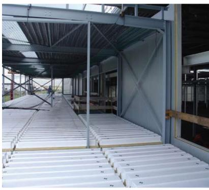
concrete floor based upon a T-beam principle (concrete rib floor). Both components, the sandwich panels and the EPS profile blocks are installed on site. The end result after fixing the reinforcement and pouring concrete is a lightweight, fully insulated floor with a large free span, small floor zone height and a smooth white under side soffit ceiling.
