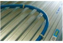
As with standard floors, ensure a 10 mm gap around the perimeter of each room by using edge strips or LEWIS® 20/15 Flanking strips.
